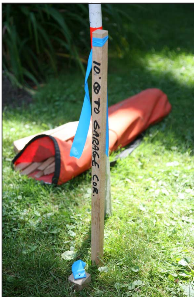
A stake is placed in the ground to define a reference distance to the back corner of the garage. The circle with an "x" in it indicates an offset.
